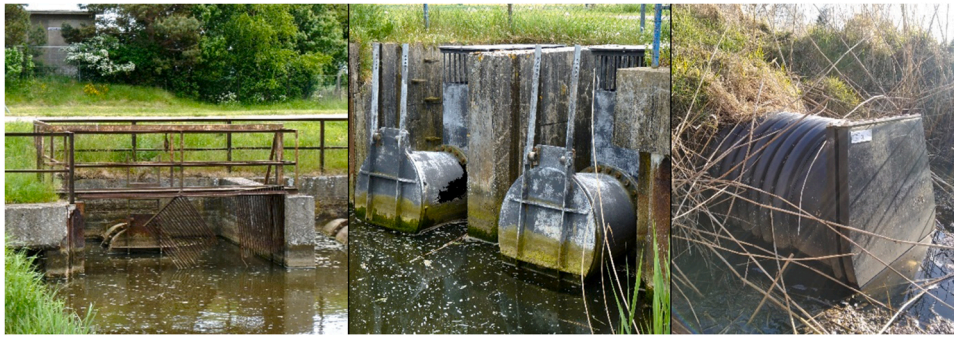
Fig. 5. Examples of barriers for directed water flow between fresh- and brackish waterbodies: Outlet of a pump shed with the main facility building in the background (left) and different types of flap gates (middle, right).
